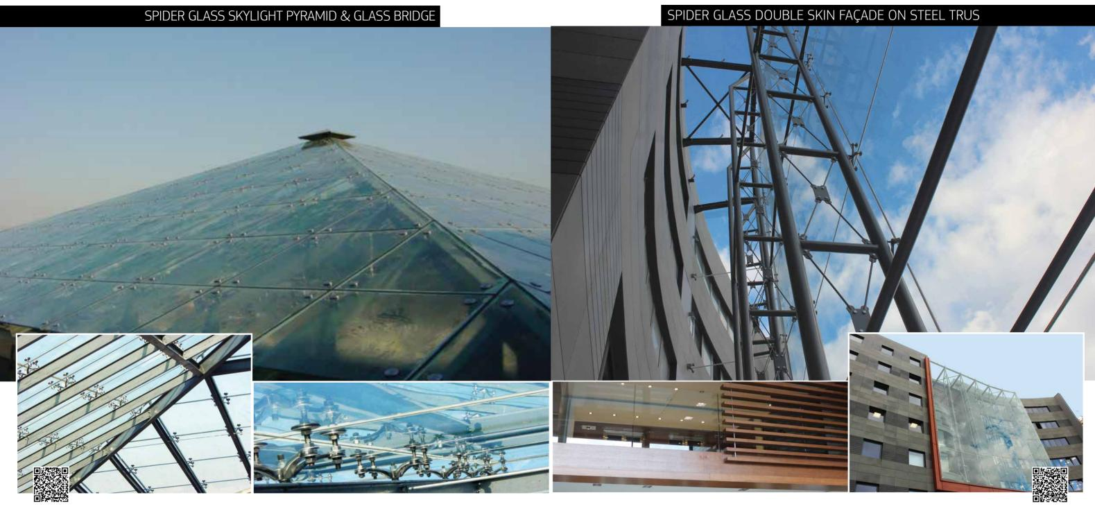
GLASSCON designed, engineered and installed an innovative glass pyramid at the top of an atrium, covering an area of 650 square meters, as well as a glass bridge for a new office building. Both systems are supported by STEEL SUB- STRUCTURE along with stainless steel 4-way spider fittings. Glass panes are made of tempered safety glass with reflective coating to provide shading while allowing daylight.
