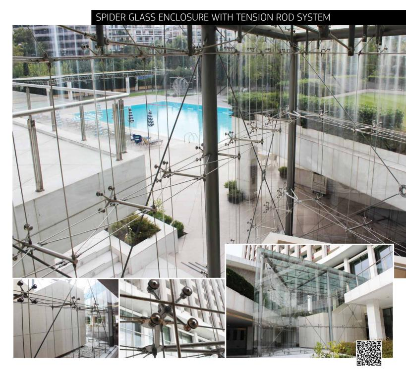
GLASSCON designed, engineered and constructed an innovative glass envelope for a staircase at a luxurious hotel. The height of this enclosure is over 12 meters. The spider glass curtain wall and roof are supported by a suspended stainless
