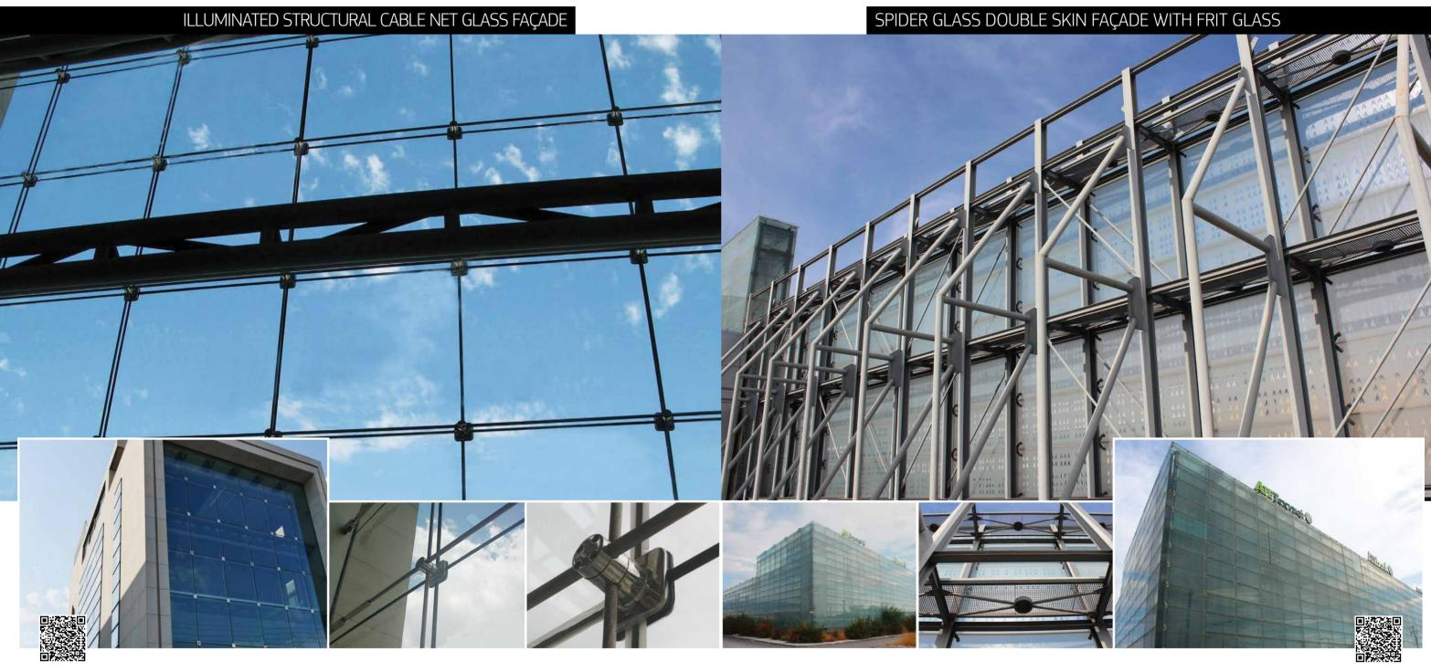
GLASSCON designed, engineered and constructed a frameless illuminated curtain wall of a total height of 25 meters for a new office building. The façade is supported by a grid of stainless steel tensioned CABLES along with custom made LED
