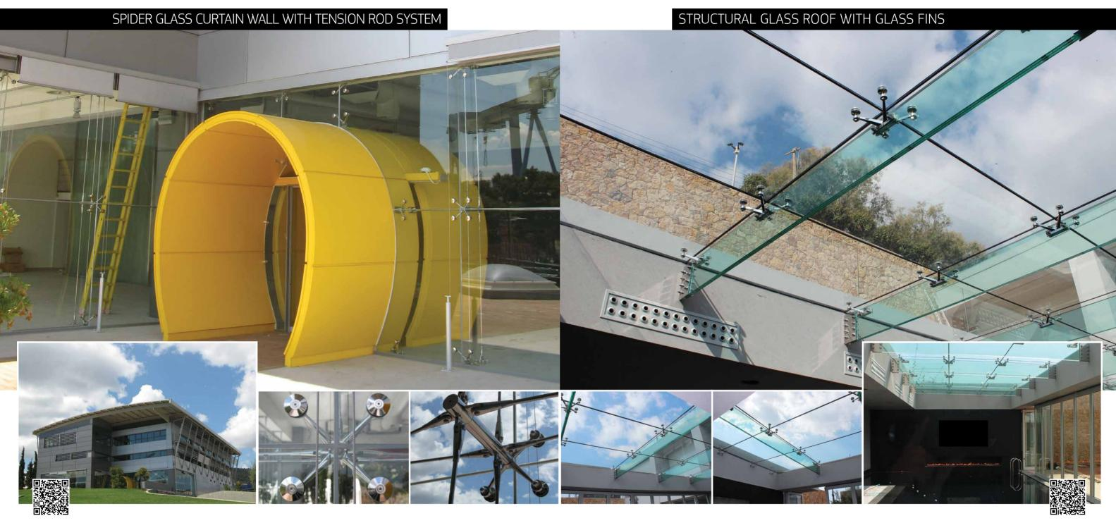
GLASSCON designed, engineered and executed the complete façade works for an office building, including motorized aluminium louvers, external brise soleil, aluminium composite panel cladding, external brise soleil and a structural glass facade. The façade is supported by a stainless steel 3D TENSION ROD SYSTEM along with pressure bars and 4-way spider glass fittings.
