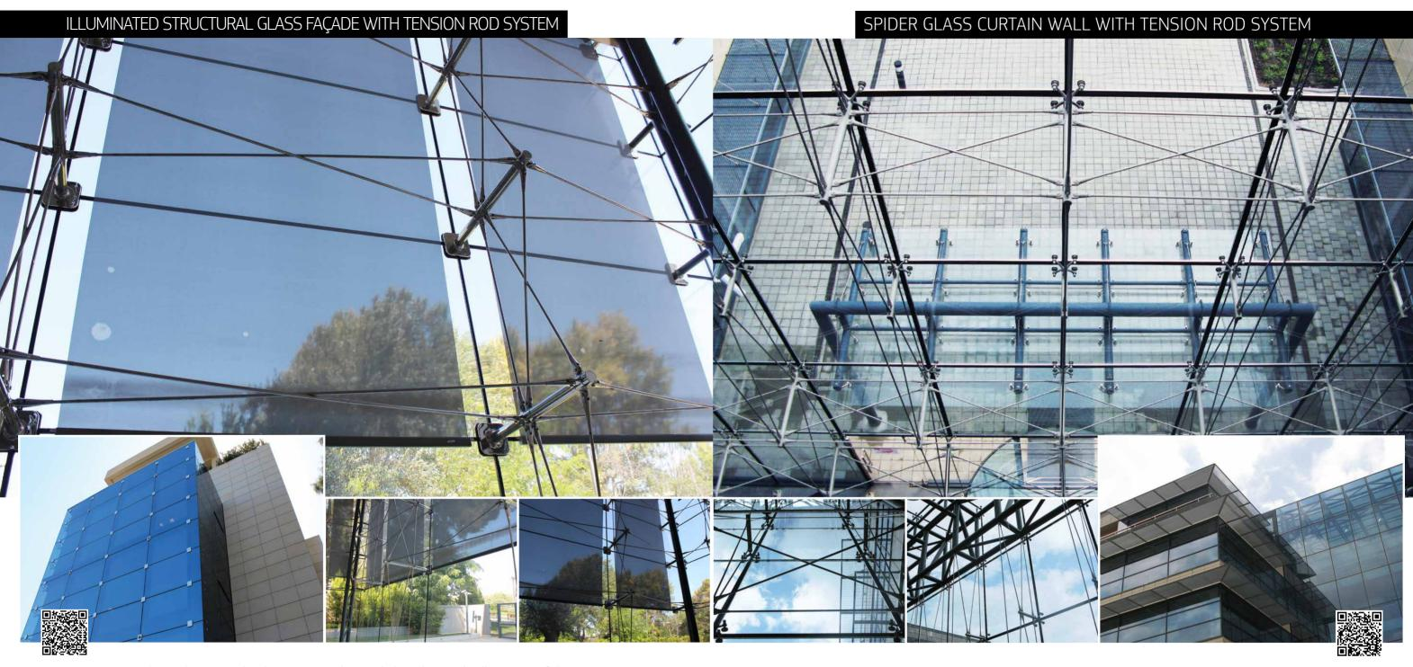
GLASSCON designed, engineered and constructed an inclined frameless illuminated curtain wall with internal shading for an office building complex. The façade is supported by a stainless steel 3D TENSION ROD SYSTEM along with pressure
