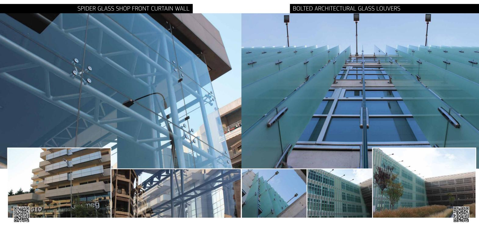
GLASSCON successfully designed, fabricated and installed a spider glass curtain wall for a SMEG front shop. The façade is supported by custom made horizontal STEEL TRUSSES, co-developed with the project architect. Glass panes
