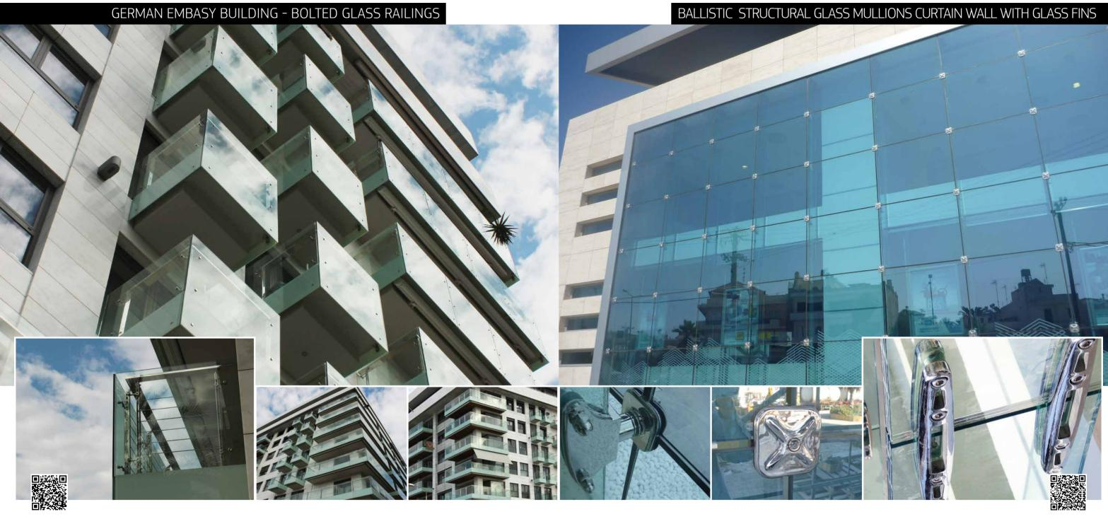
GLASSCON successfully designed, fabricated and installed a building envelope for a German Embassy building, which includes external STAINLESS STEEL & GLASS RAILS. All fittings and rails are made of high quality 316L mirror
