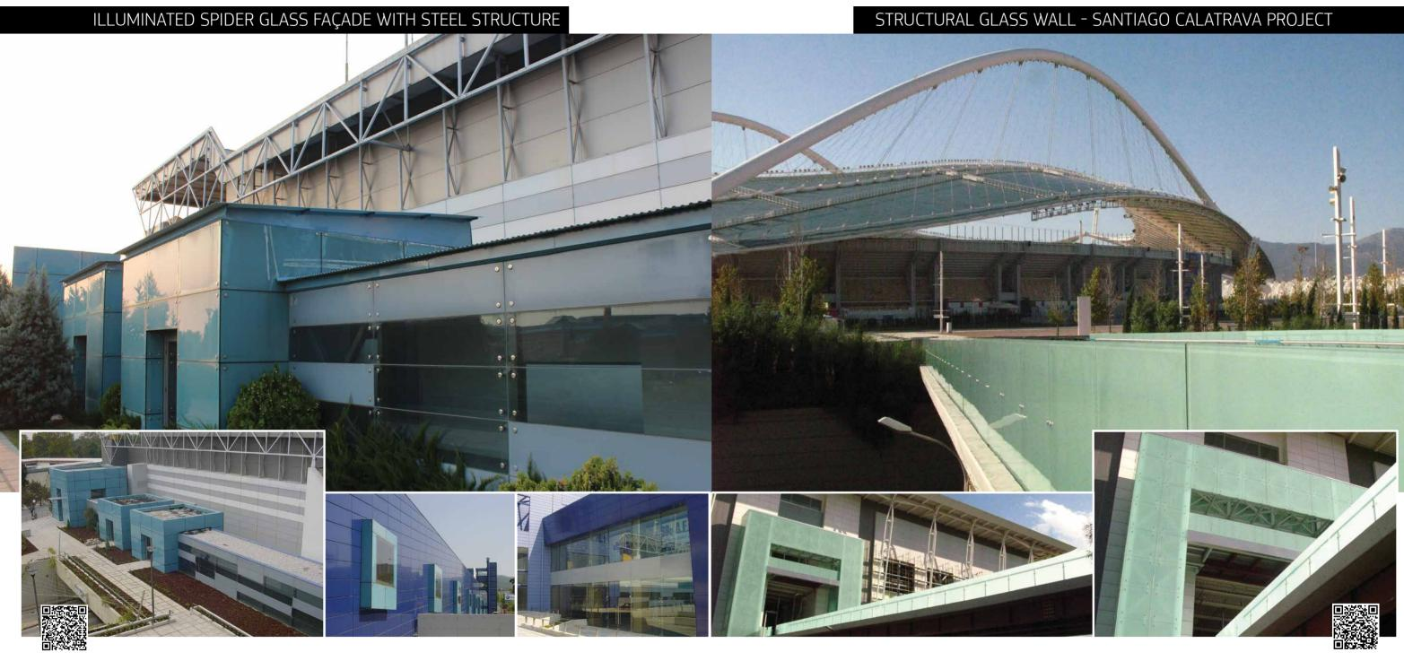
GLASSCON designed, engineered and executed various façade works for an exhibition center including an illuminated structural glazing curtain wall, aluminium composite panels cladding, glass
