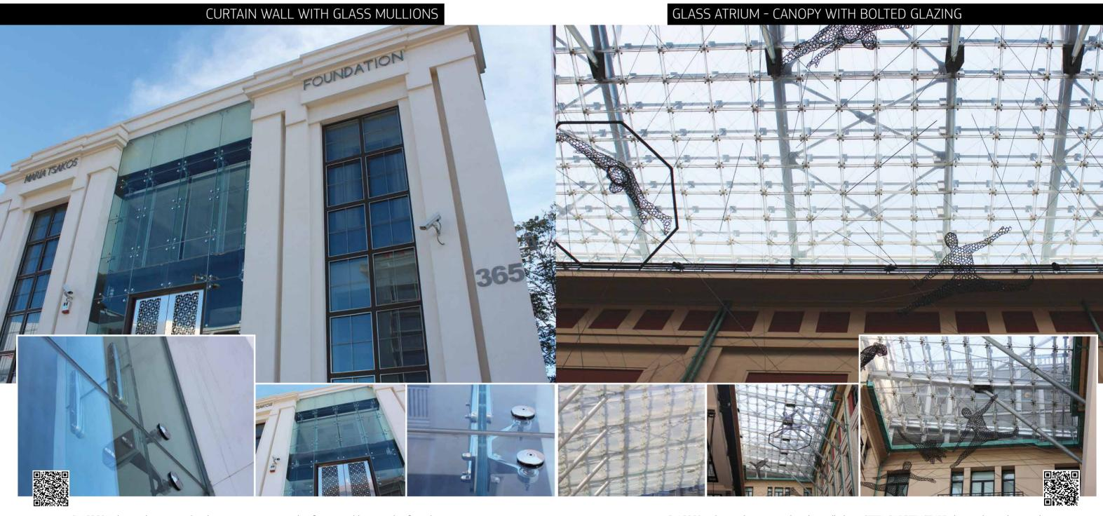
GLASSCON designed, engineered and constructed a structural curtain wall for an iconic building facade. The façade is almost 100 % transparent as it is supported by GLASS MULLIONS along with 4-way spider glass fittings. Glass mullions
