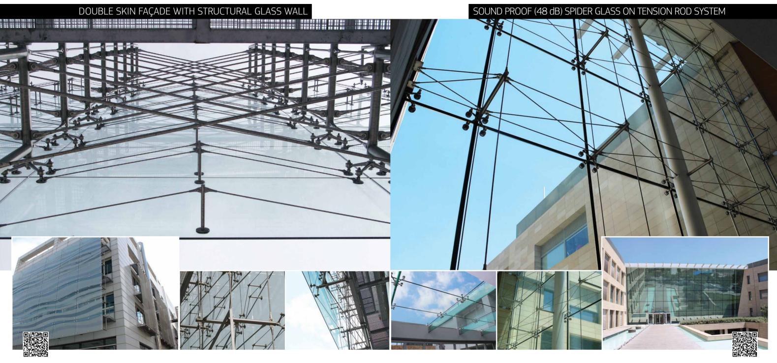
GLASSCON designed, engineered and executed the complete façade works for an office building, including aluminium solar shades, cladding, inox meshes and point fixed second skin glass façade. The double skin glass façade is supported by a stainless steel 3D TENSION ROD SYSTEM com-
