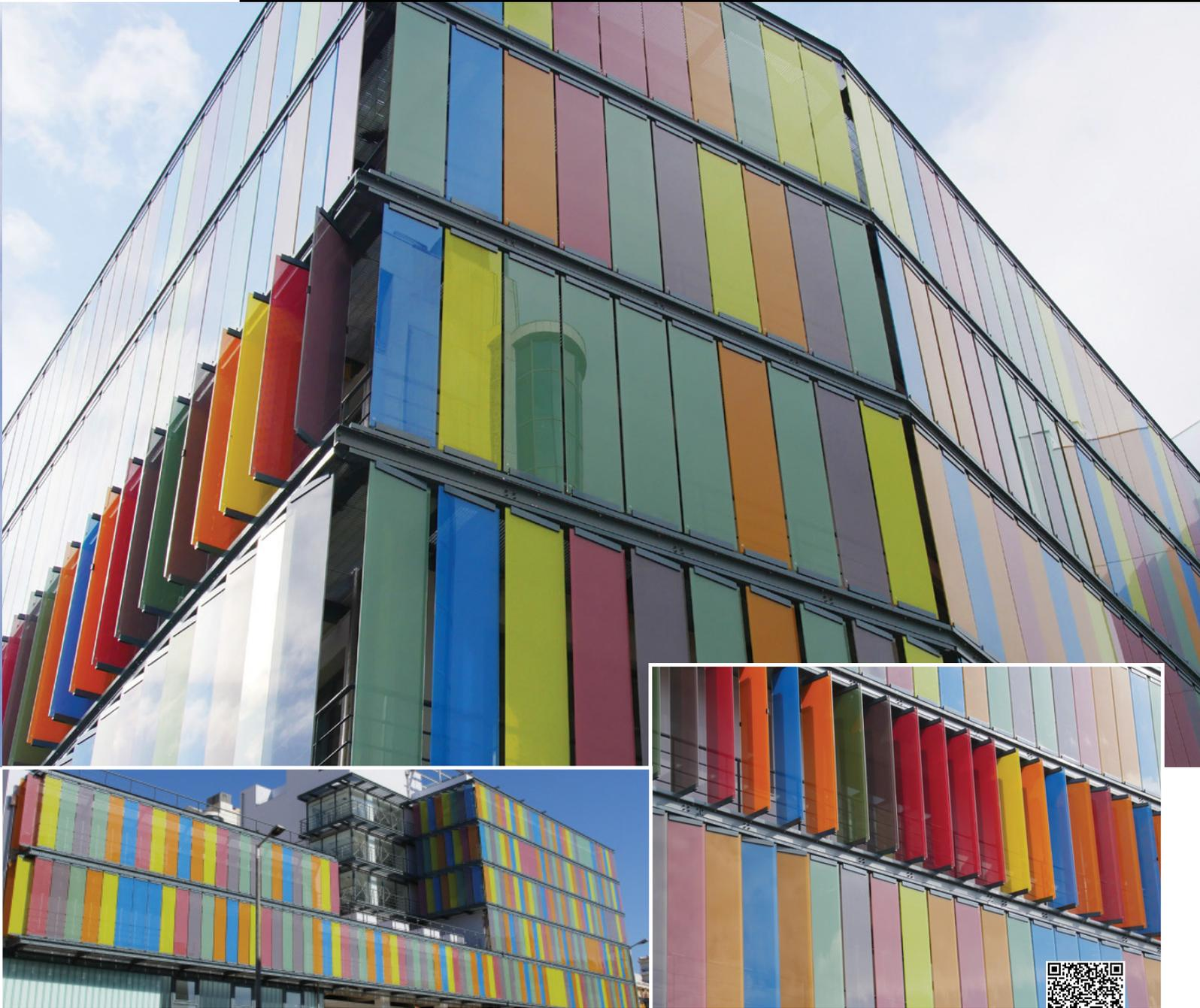
GLASSCON developed, fabricated and installed a stunning solar shading system as a building envelope. Our SILK PRINTED GLASS LOUVERS feature six stimulating colors providing 20% transparency and are fitted with special stainless steel IPS 65 ELERO linear actuators. Louvers ro-
