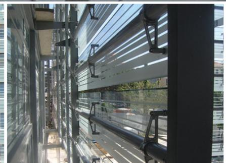
GLASSCON designed, fabricated and installed an innovative second skin shading system for a bank branch with MOVABLE GLASS LOUVERS operating fully automated. The glass louvers carry special ceramic printing technology to create the desired design pattern and provide efficient shading.
