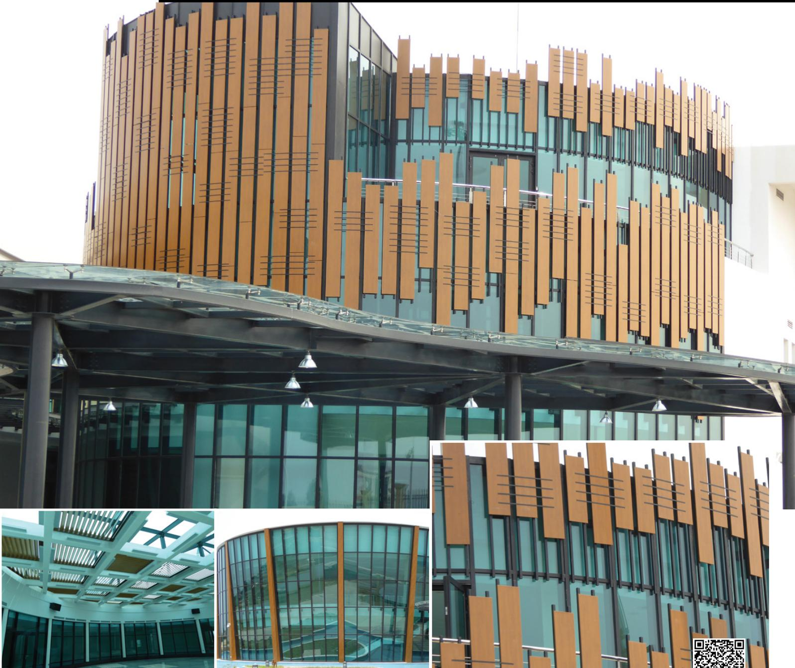
GLASSCON successfully executed the complete façade works for the Presidential Conference Centre located at Brazzaville International Airport of Congo, which was engineered by LUFTHANSA CONSULTING. Façade works include honeycomb shading panels as well as ballistic curtain walls,
