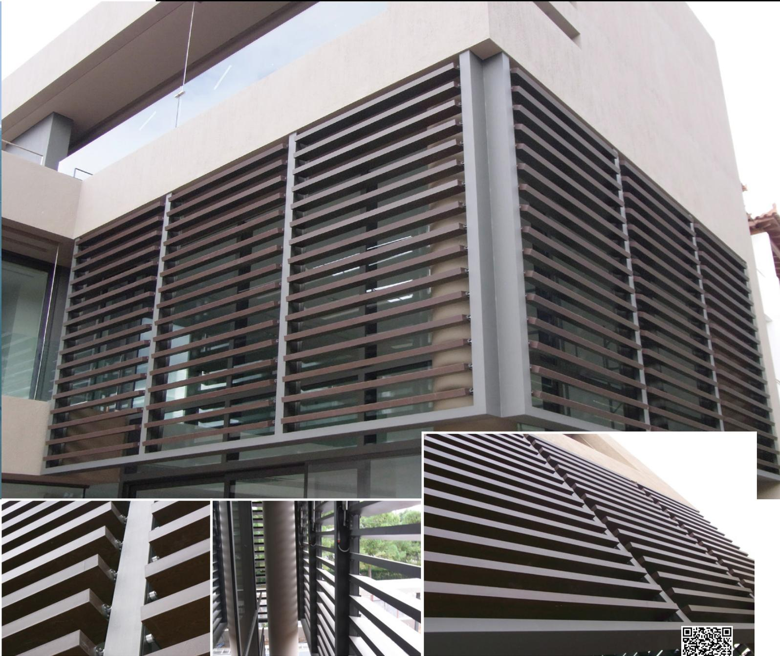
GLASSCON designed, developed and installed an external architectural motorized HPL SOLAR LOUVERS with a wood finish. The selected certified material is extremely weather and UV resistant, making it a low maintenance eco-friendly solution for outdoor small scale
