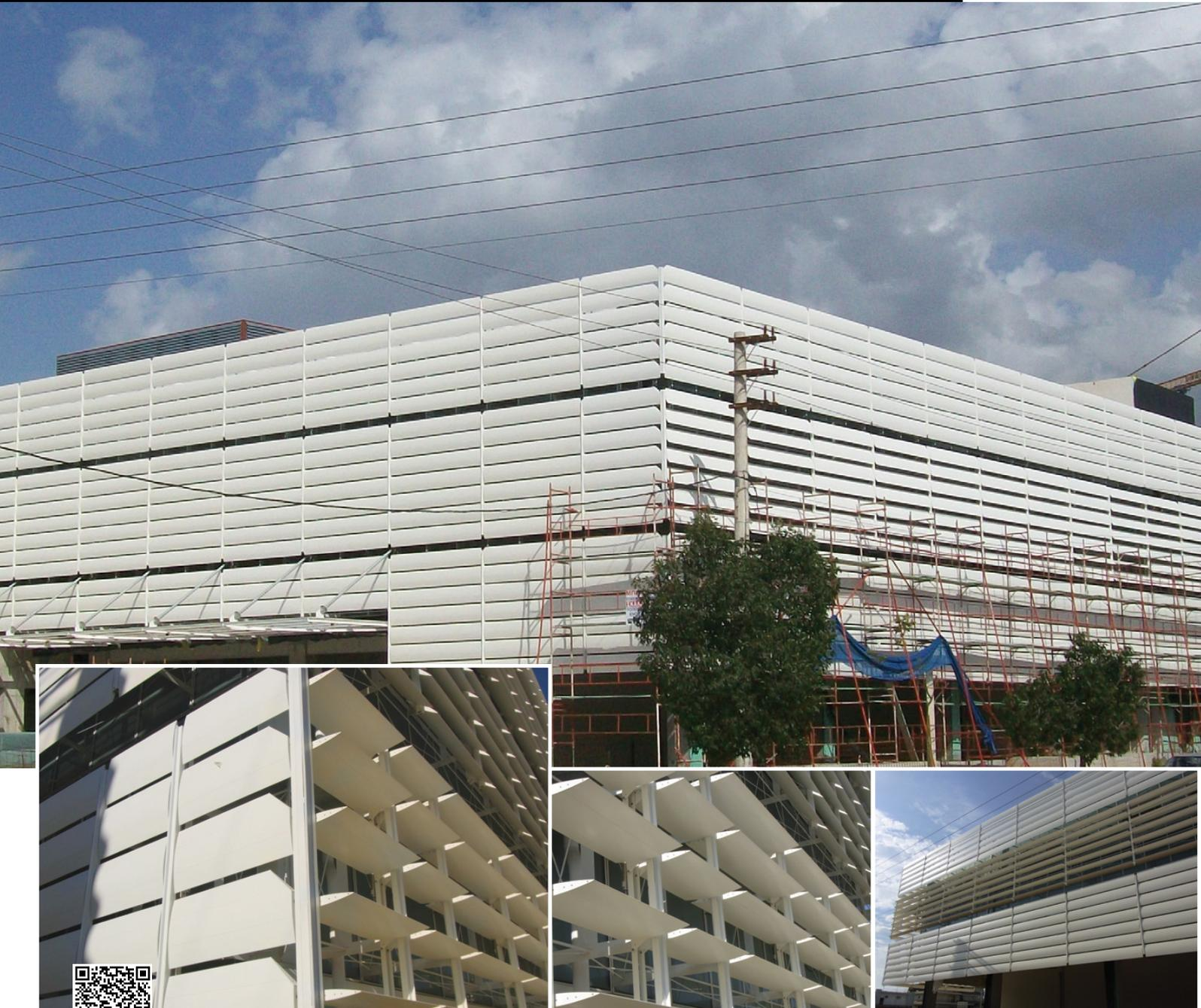
GLASSCON designed, engineered and constructed a fully motorized external shading system with ALUMINIUM AIRFOILS for a telecommunications office building. The selected material has an aero blade shape and is certified for its rigidity and durability. According to the solar shading study results, the whole façade had to be totally
