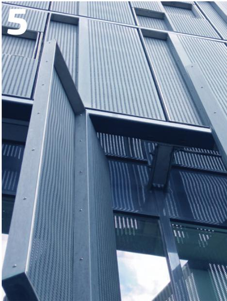
**METAL LOUVERS type “GL/ML” (SPECIAL / PERFORATED / EMBOSSED)**
