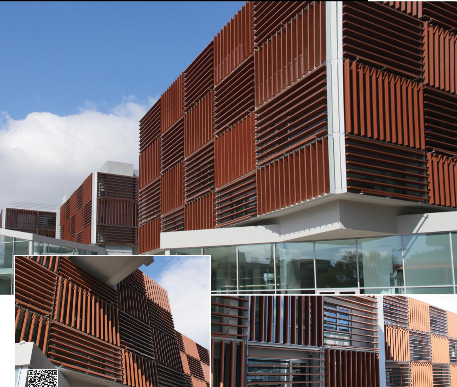
GLASSCON was involved in the rehabilitation works of an office building complex, including the design, engineering, fabrication and installation of an architectural second skin which contributed the most to building's LEED Gold certification. The kinetic solar shading system combines solar gain
