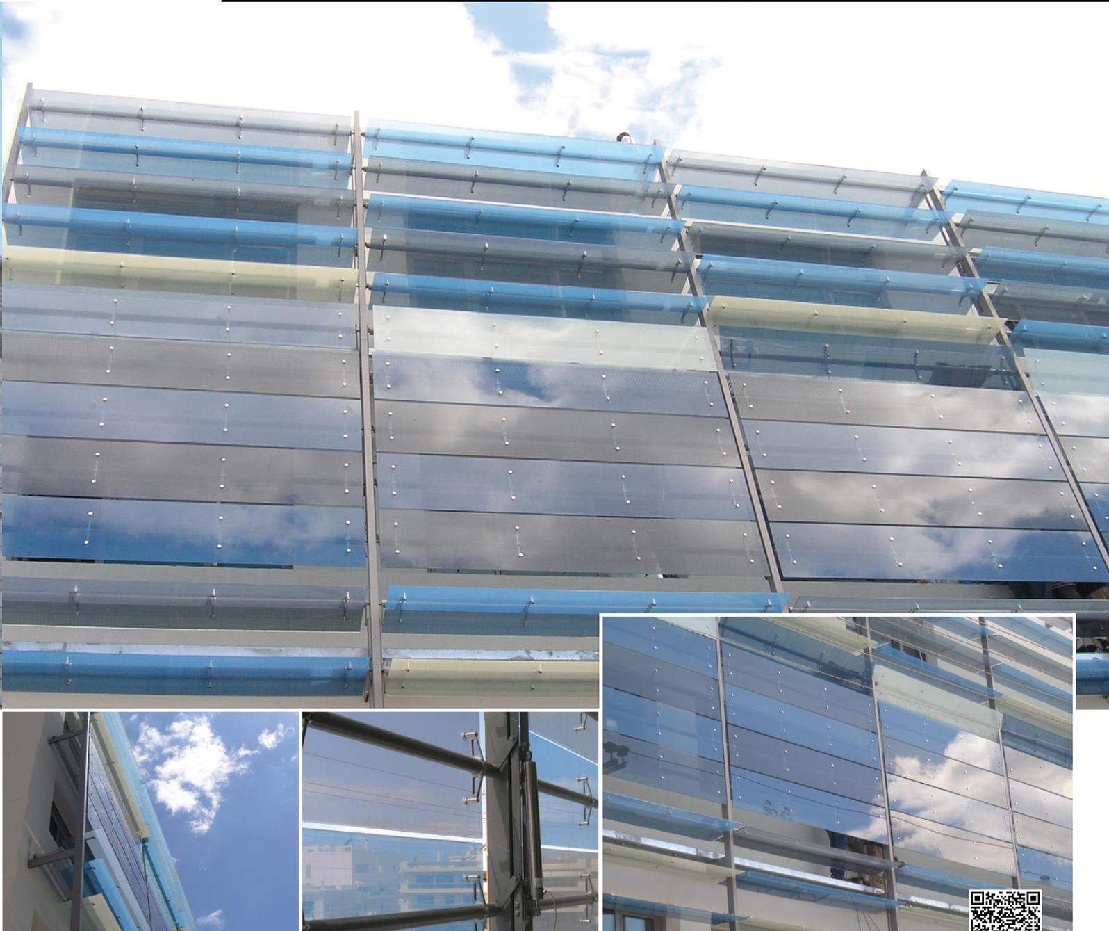
GLASSCON designed, fabricated and installed an innovative second skin shading system for an eye clinic with MOVABLE GLASS LOUVERS operating fully automated. The glass louvers carry silk printing to create the desired transparency and provide efficient shading. Glass used is tempered
