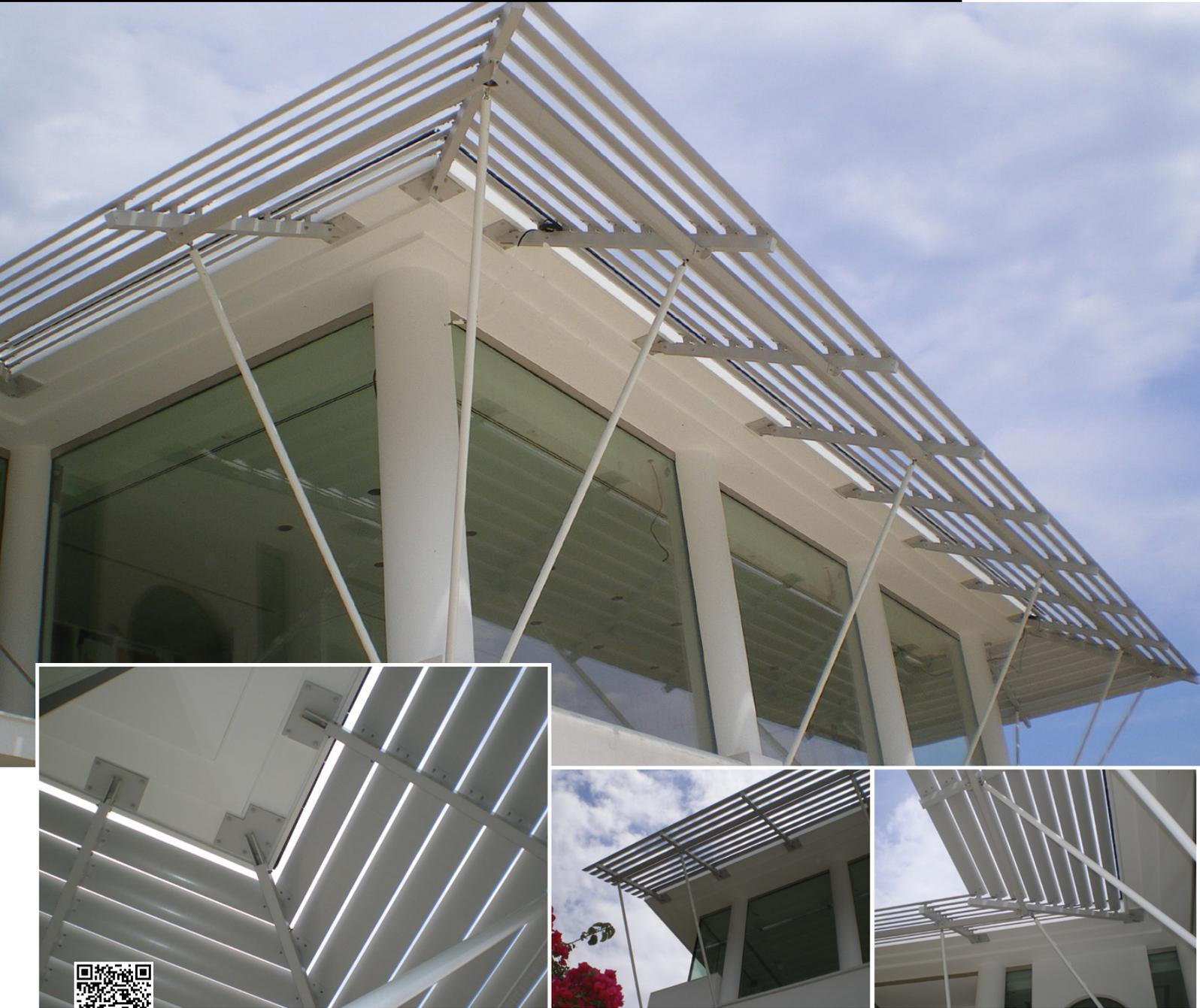
GLASSCON designed, engineered and constructed a brise soleil cantilever system for a country house with integrated FIXED ALUMINIUM BLADES. After comprehensive shading study, the selected system allows undisturbed view from the interior of the building, whilst providing ef-
